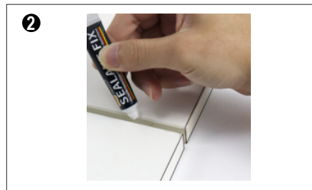
Filled with adhesive in the recessed groove
